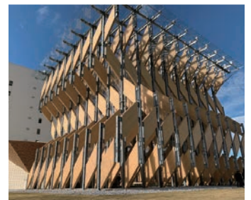
Traditional wooden frame construction + CLT
